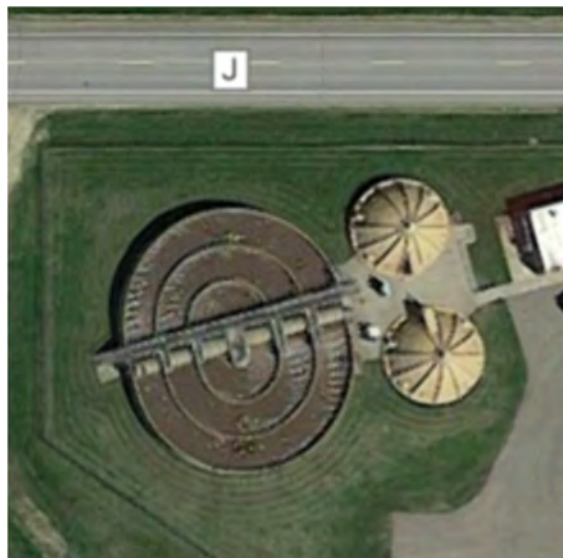
Figure 1 – Existing Oxidation Ditch and Clarifiers
